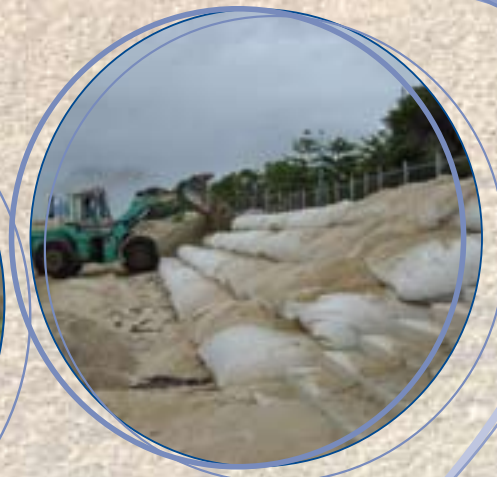
Rockingham Foreshore, WESTERN AUSTRALIA
