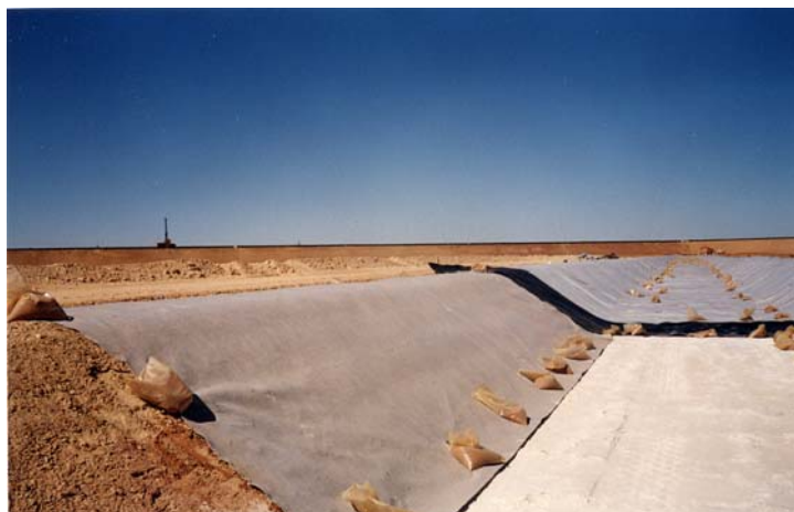
Decant drainage channel continued at a depth of 3 metres (gravity feed)
