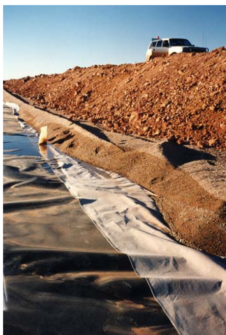
Decant causeway with Bidim geotextile protection layer over HDPE liner (A44)
