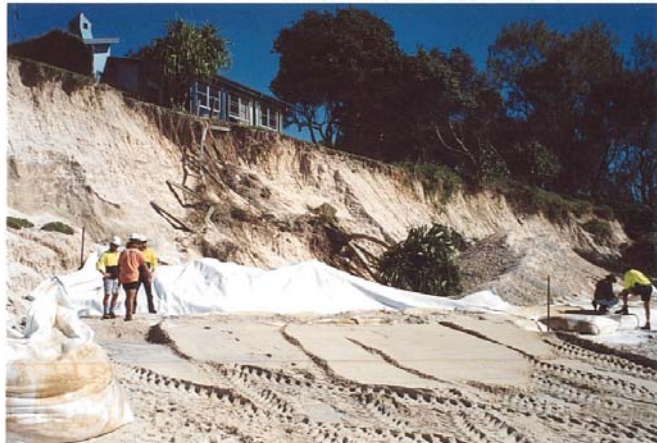
House in danger July 1999
